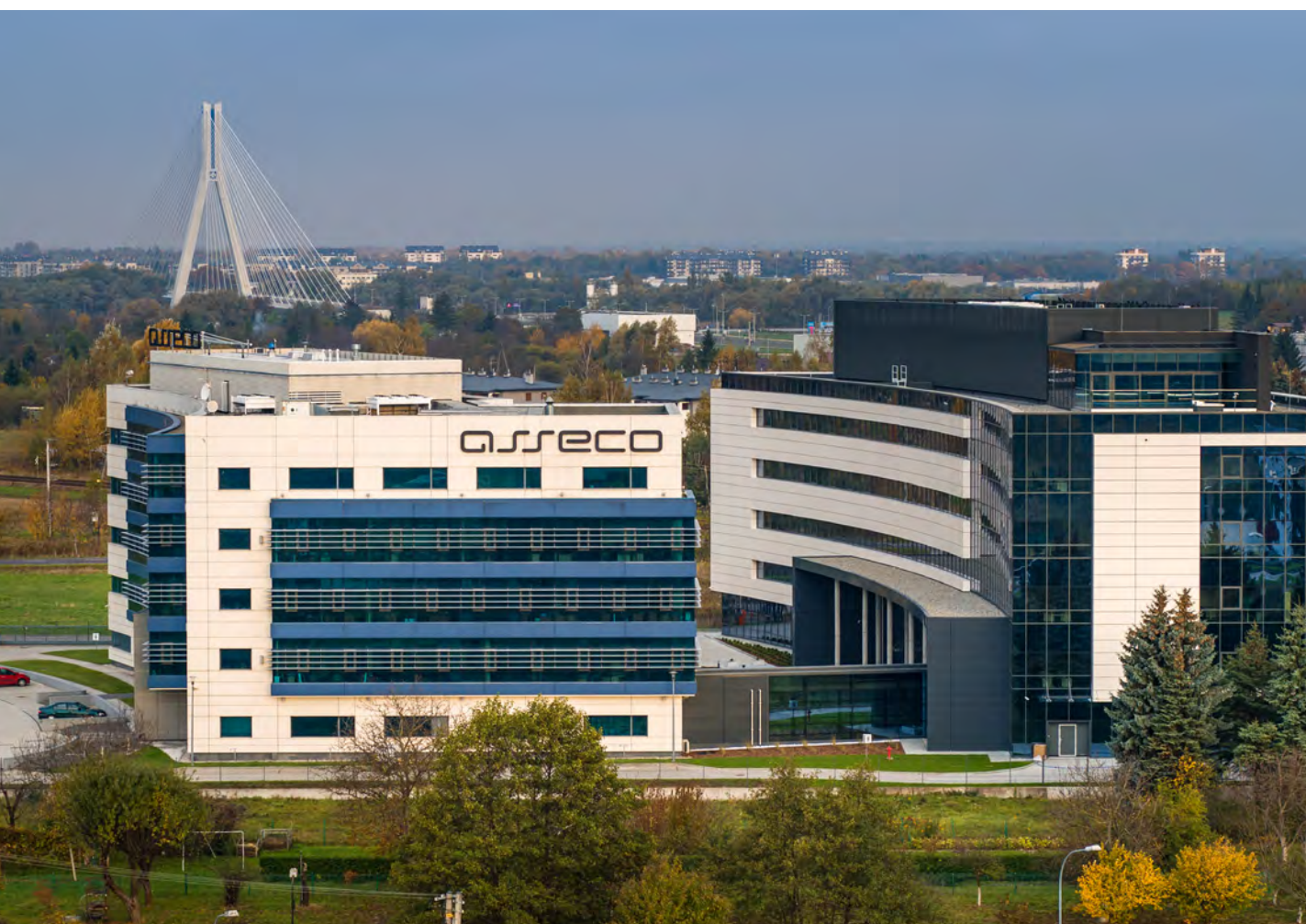
Asseco Poland Headquarters, source: City Office of Rzeszów
